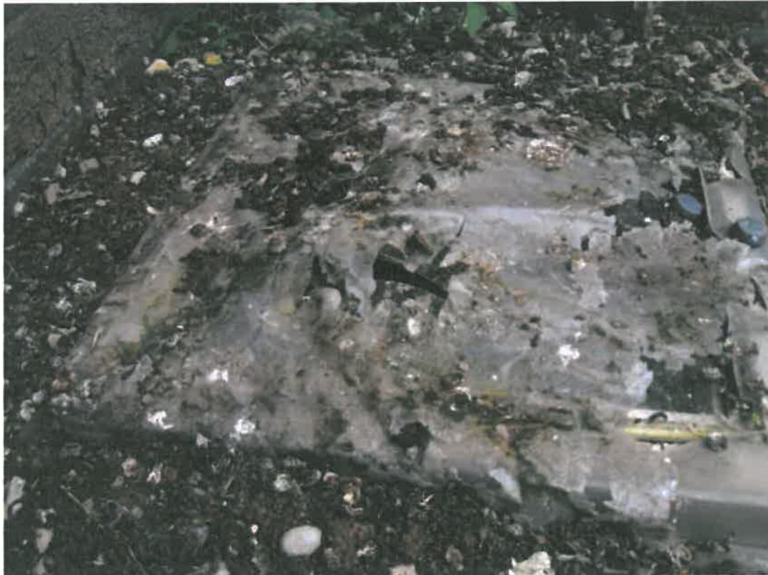
Foto 95 Gebroken lichtkeepel.
